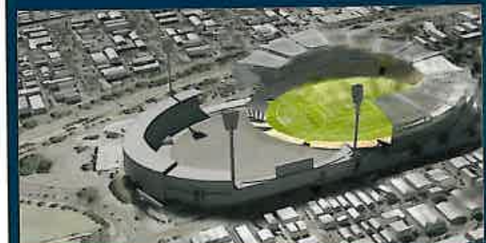
Subiaco Stadium - Stage 2
